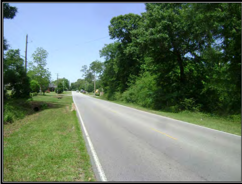
West Ten Mile Road, subject lots on right, western view, 04/28/2011
